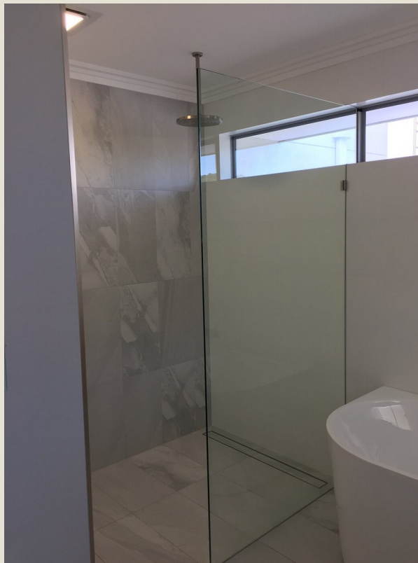
Bright, contemporary finishes from a recent project.
